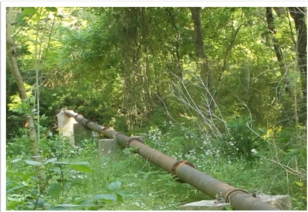
FIGURE 4: HOWEL MILL OUTFALL AERIAL SEWER
