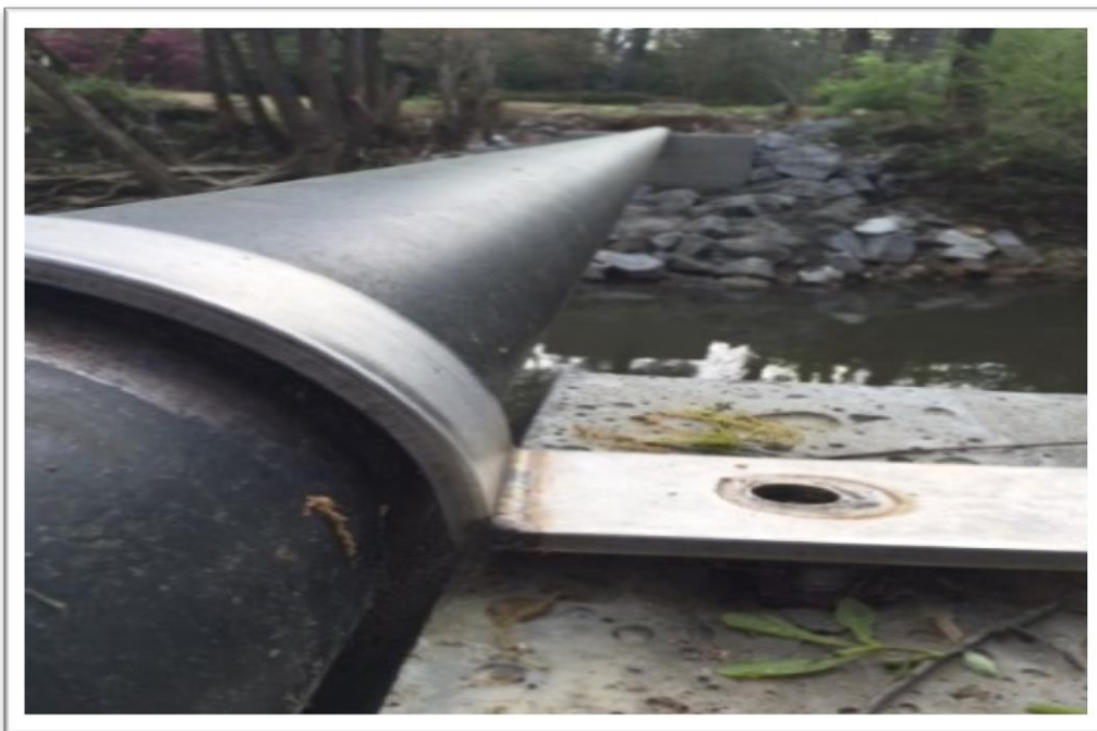
FIGURE 8: OLDFIELD OUTFALL AERIAL SEWER (COMPROMISED PIPE STRAP)
