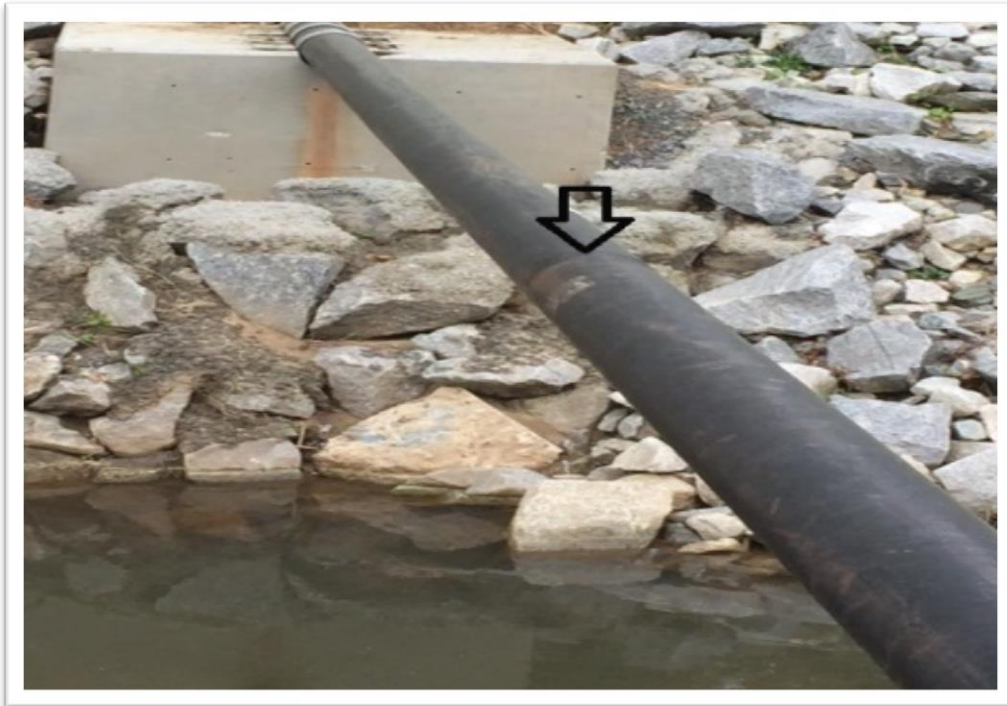
FIGURE 7: OLDFIELD OUTFALL AERIAL SEWER (EXPOSED PIPE SEAM)
