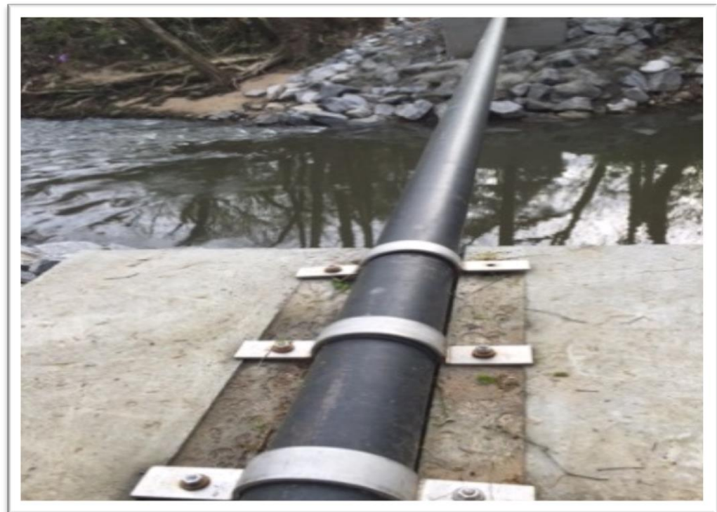
FIGURE 6: OLDFIELD OUTFALL AERIAL SEWER
