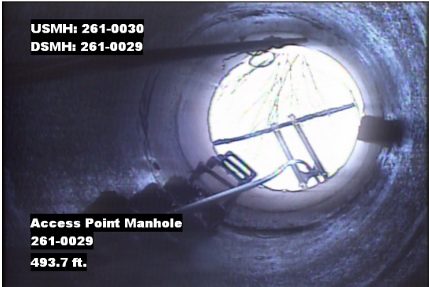
Photo: 261-0030_261-0029_AMH_493.7.jpg, VCR No.: 1 493.7FT, Manhole
