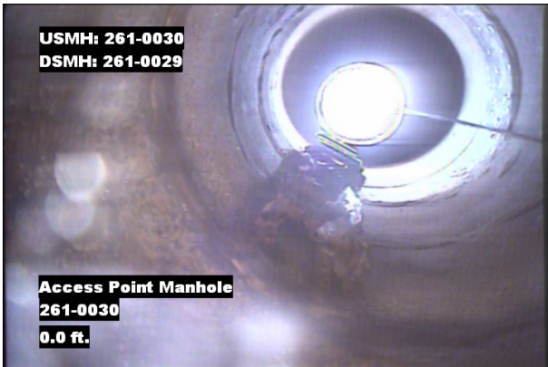
Photo: 261-0030_261-0029_AMH_0.0.jpg, VCR No.: 1 0FT, Manhole
