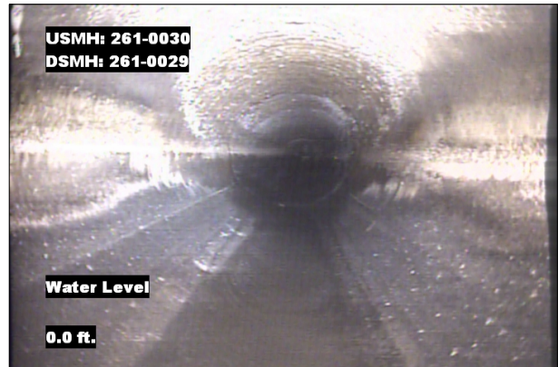
Photo: 261-0030_261-0029_MWL_0.0.jpg, VCR No.: 1 0FT, Water Level, 5% of cross sectional area
