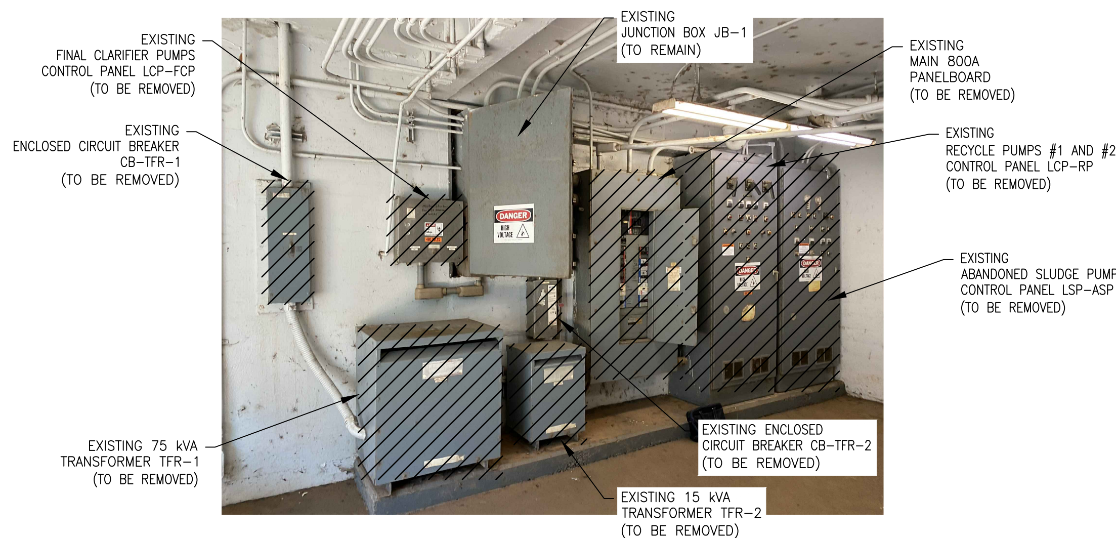
3 EXISTING ELECTRICAL EQUIPMENT (DEMOLITION SCOPE)
