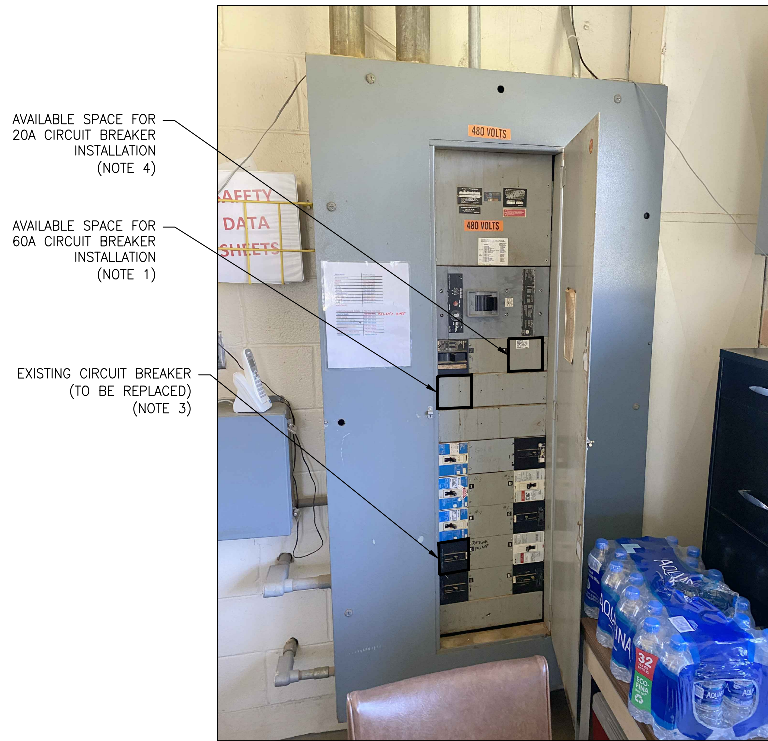
2 EXISTING PANELBOARD PP-1 (PROPOSED MODIFICATIONS) (WESTINGHOUSE PANELBOARD, CAT# AT41254 IT1; TYPE CDP)
