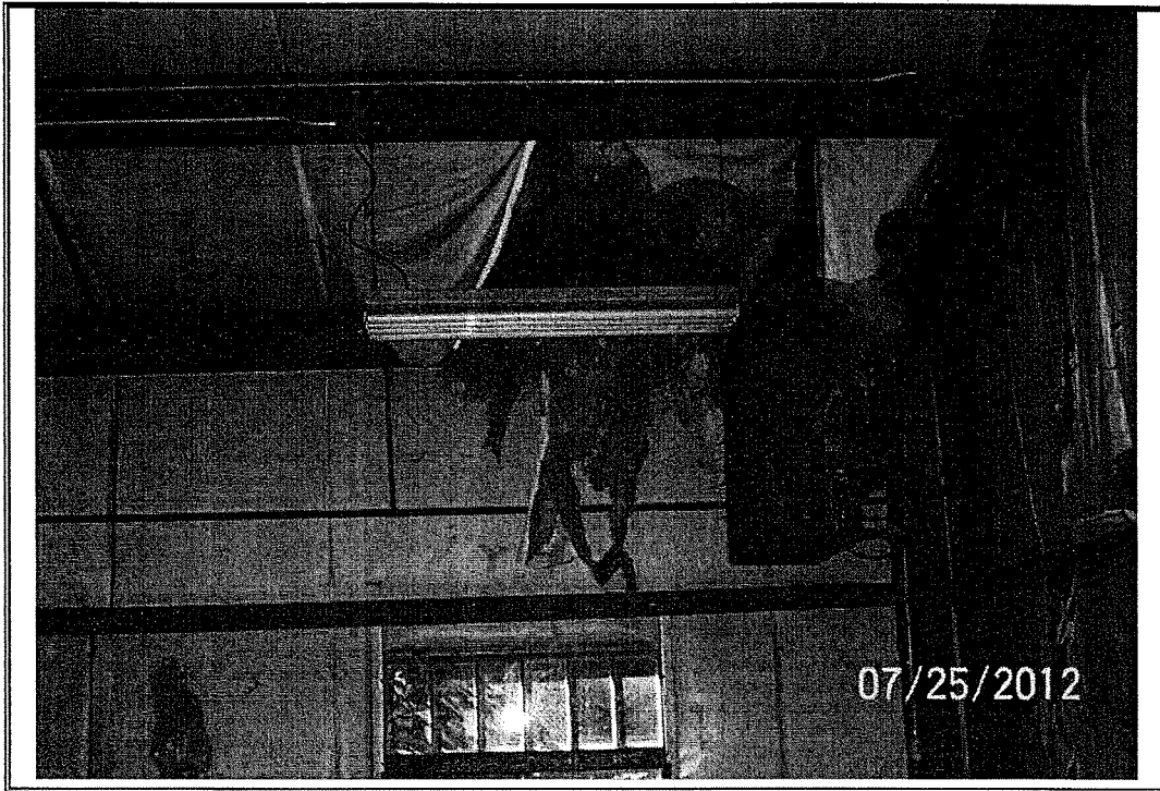
Photo # 5: View of insulation in M Bid. (ND)
