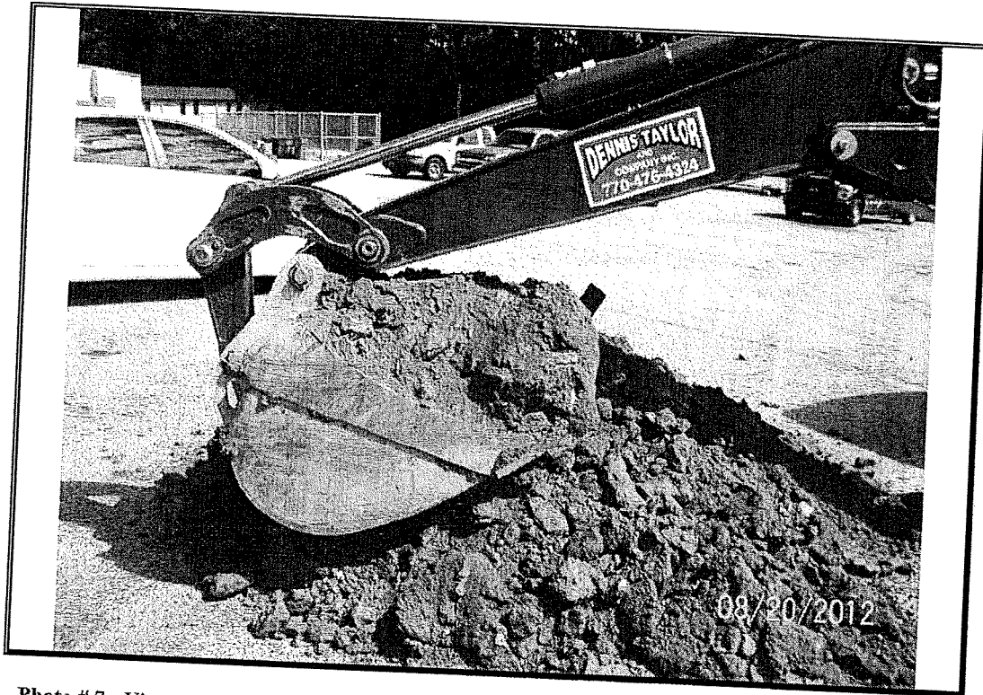
Photo # 7: View of top 2' of soils removed from test pit T-5.
