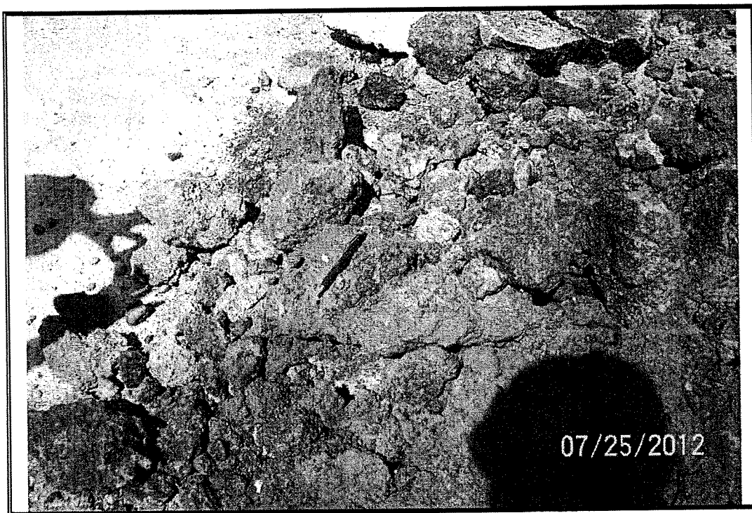
Photo # 6: View of "slag like" materials removed from TP-4.
