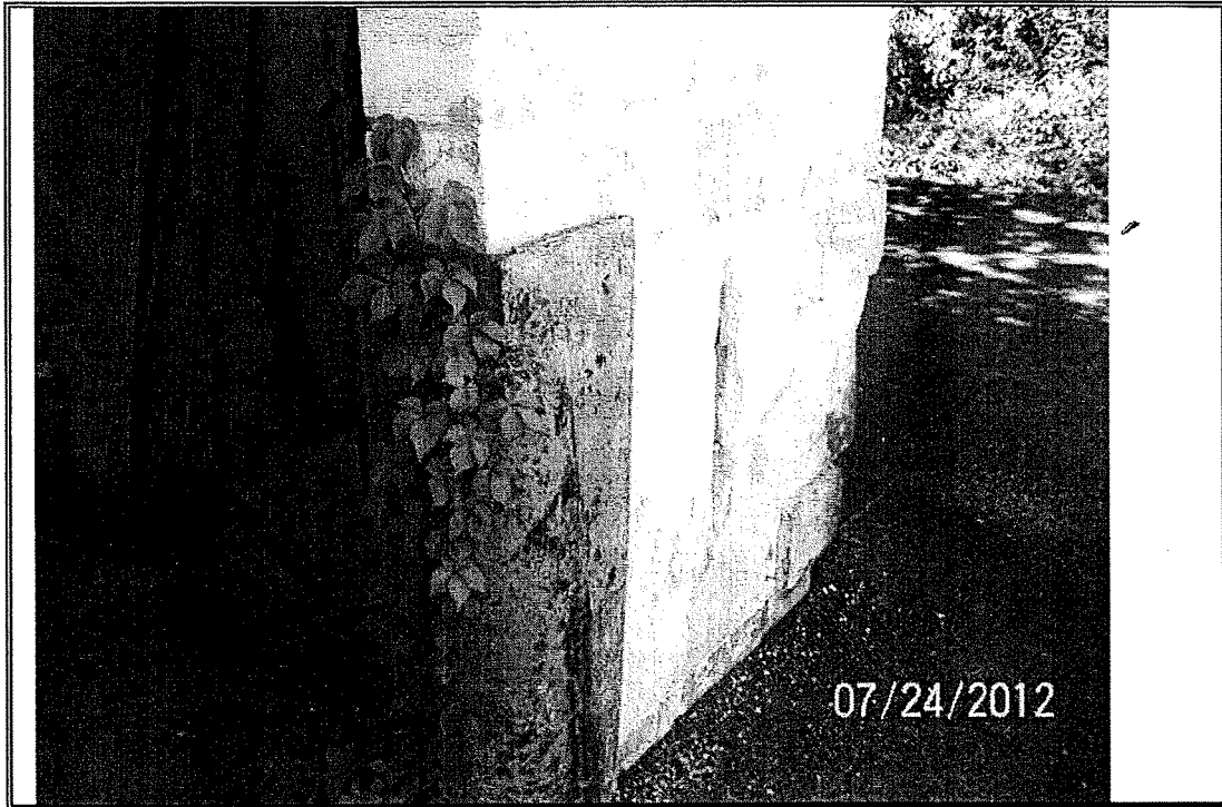
Photo # 7: View of the car bumper (red) and the exterior wall (white) both found to contain lead at 15.4 % and 1.3 %, respectively.
