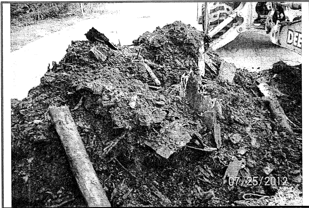
Photo # 2: Remaining soils/debris excavated from TP-1.
