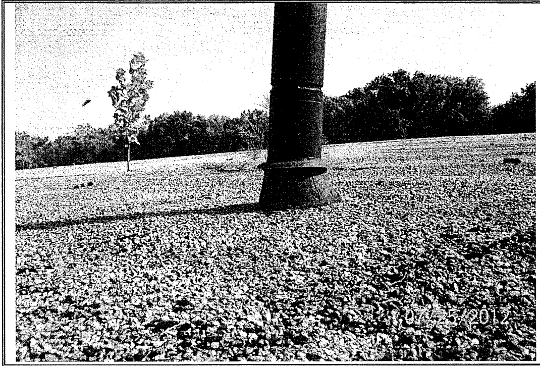
Photo # 3: .View of vent pipe/roof penetration mastic/tar on C Bld. (20 % CH)
