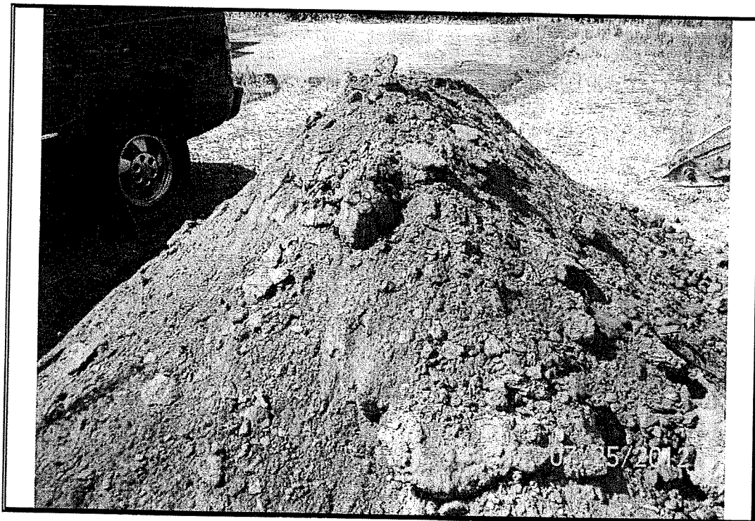
Photo # 4: .View of soils excavated from TP-3.
