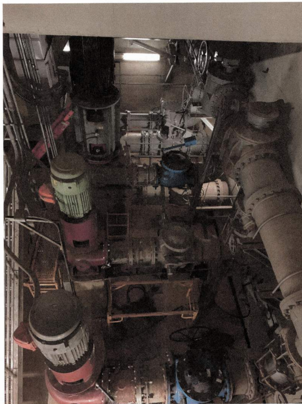
PUMP GALLERY - NORTH VIEW
