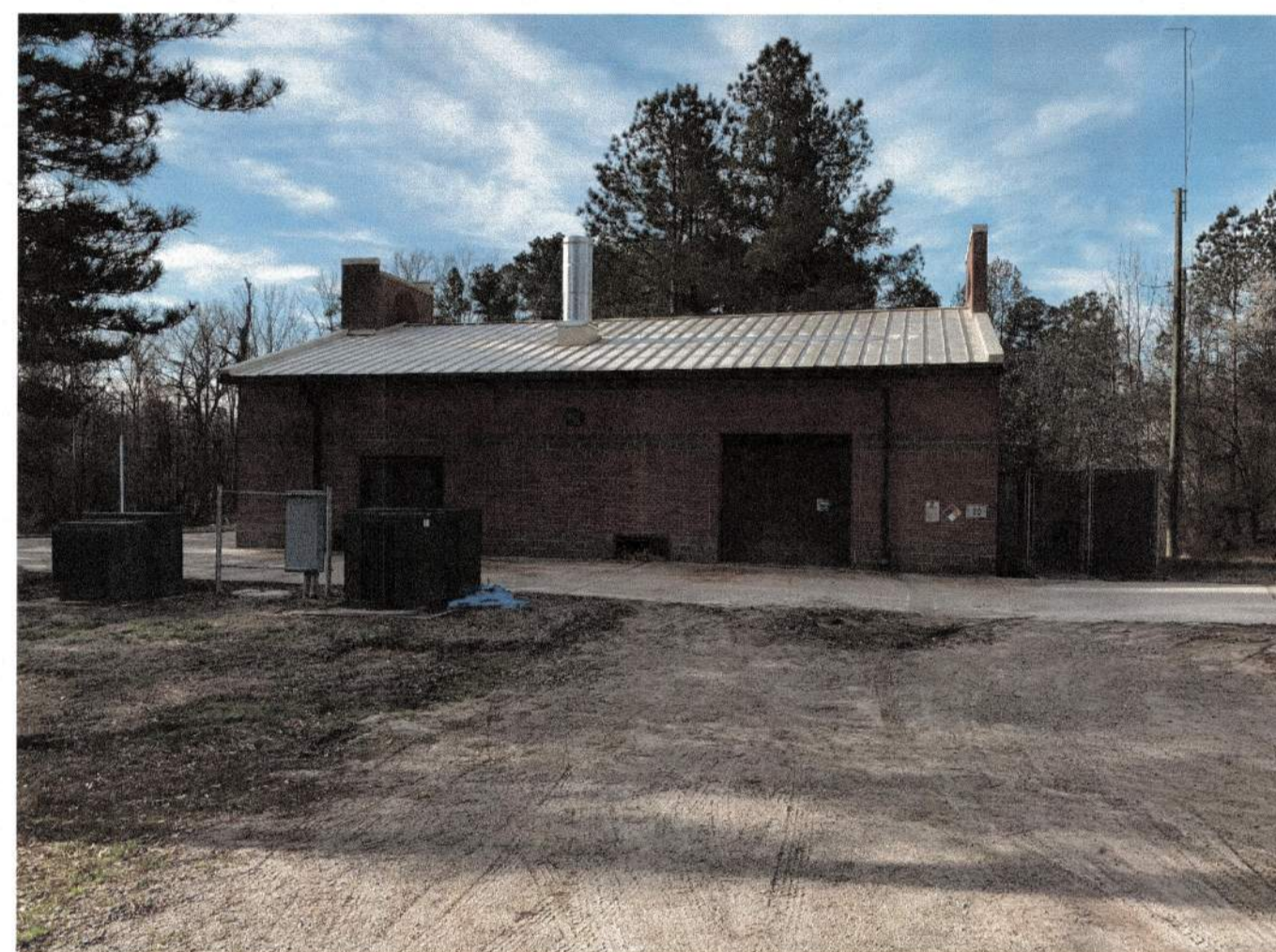
SUPERSTRUCTURE - NORTH ELEVATION
