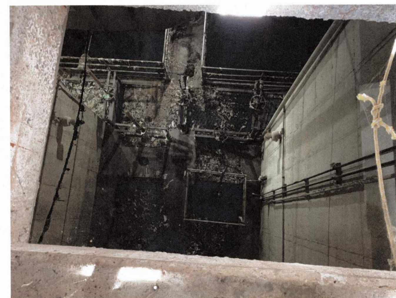
WET WELL - EAST END
