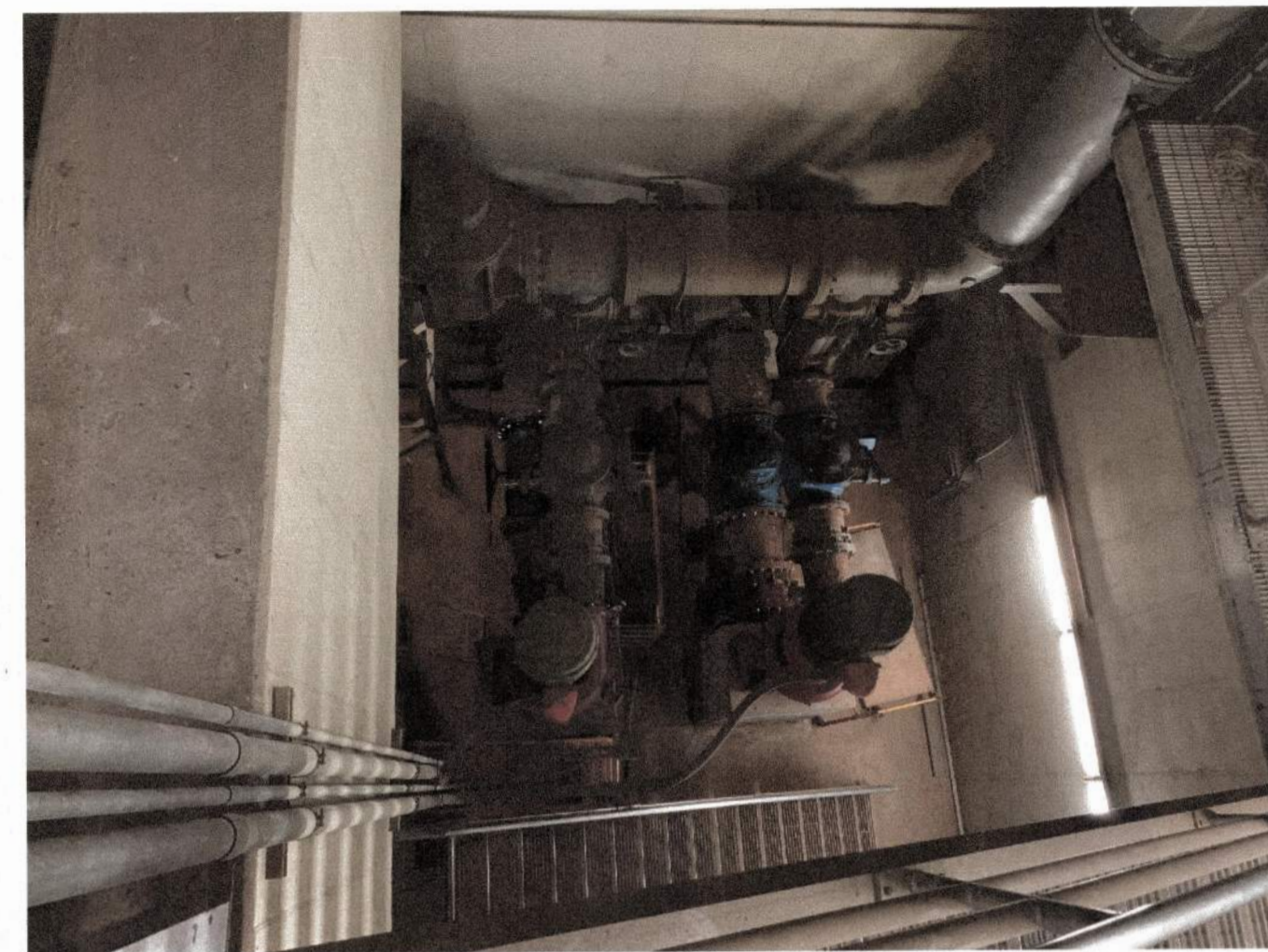
PUMP GALLERY - SOUTH VIEW
