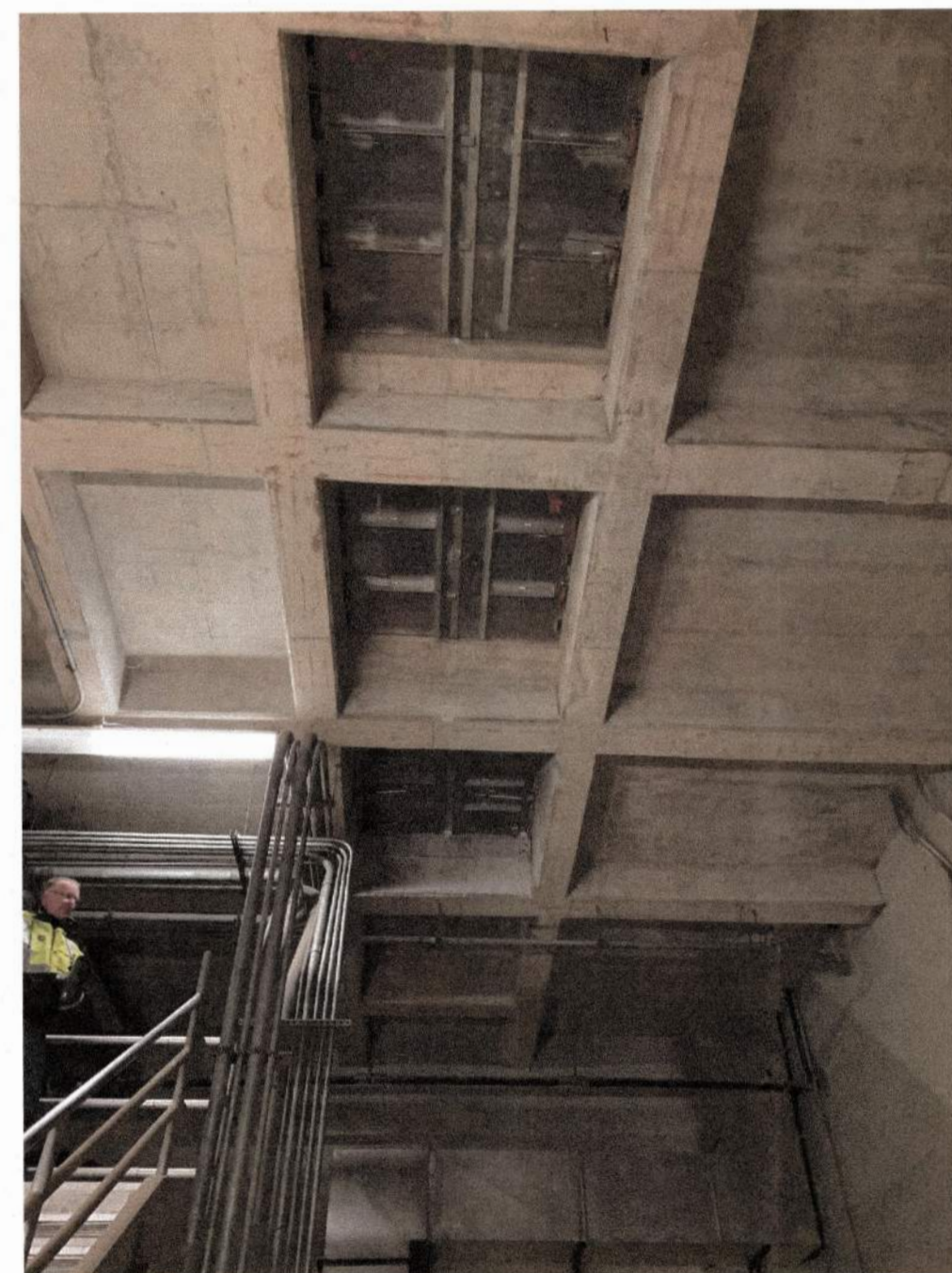
PUMP GALLERY - CEILING
