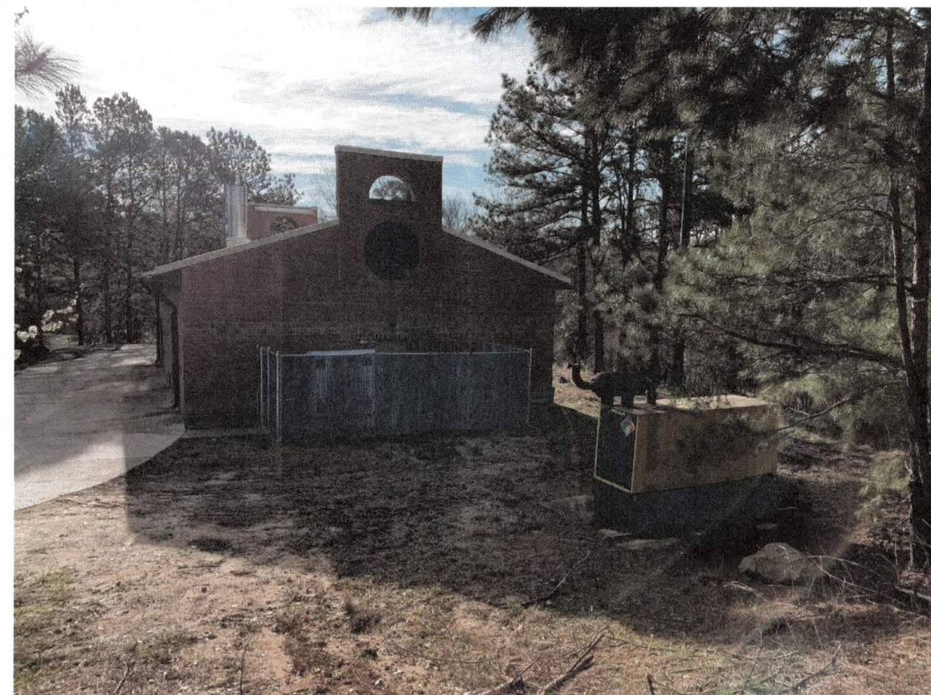
SUPERSTRUCTURE - WEST ELEVATION
