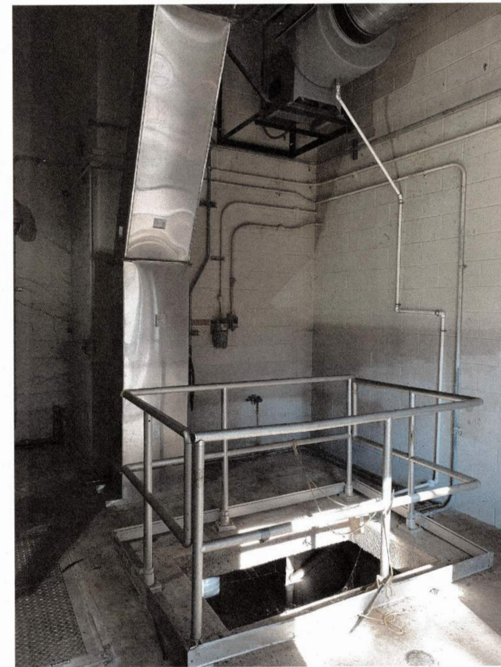
WET WELL - UPPER LEVEL
