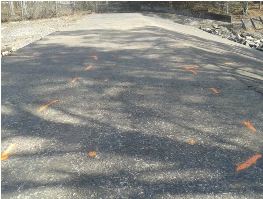
Figure 7: View the northwest anomalous area along the top of the dam.
