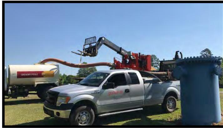
Figure 4.2: Pump connected to water truck and pig launcher
