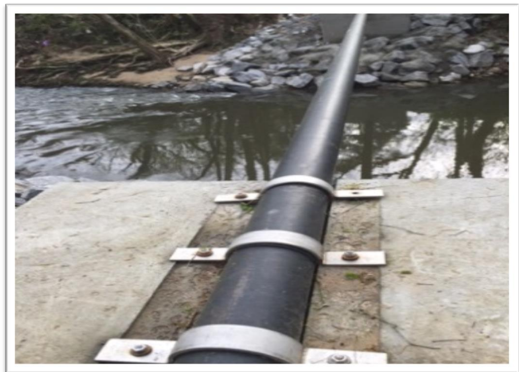
FIGURE 6: OLDFIELD OUTFALL AERIAL SEWER
