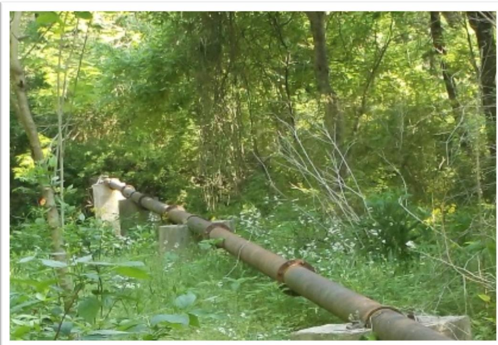
FIGURE 4: HOWEL MILL OUTFALL AERIAL SEWER
