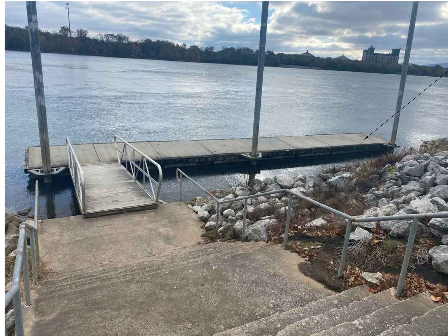
CONCRETE FLOATING DOCK MODIFICATIONS
