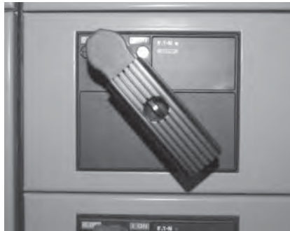
Circuit Breaker Handle Mechanism
