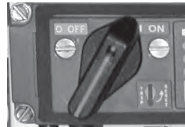
Circuit Breaker Handle Mechanism
