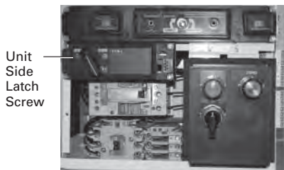
Freedom FlashGard Unit Wrapper Side Latch
