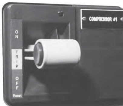
Circuit Breaker Handle Mechanism
