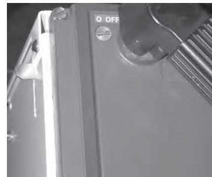
Unit Insertion Interlock
