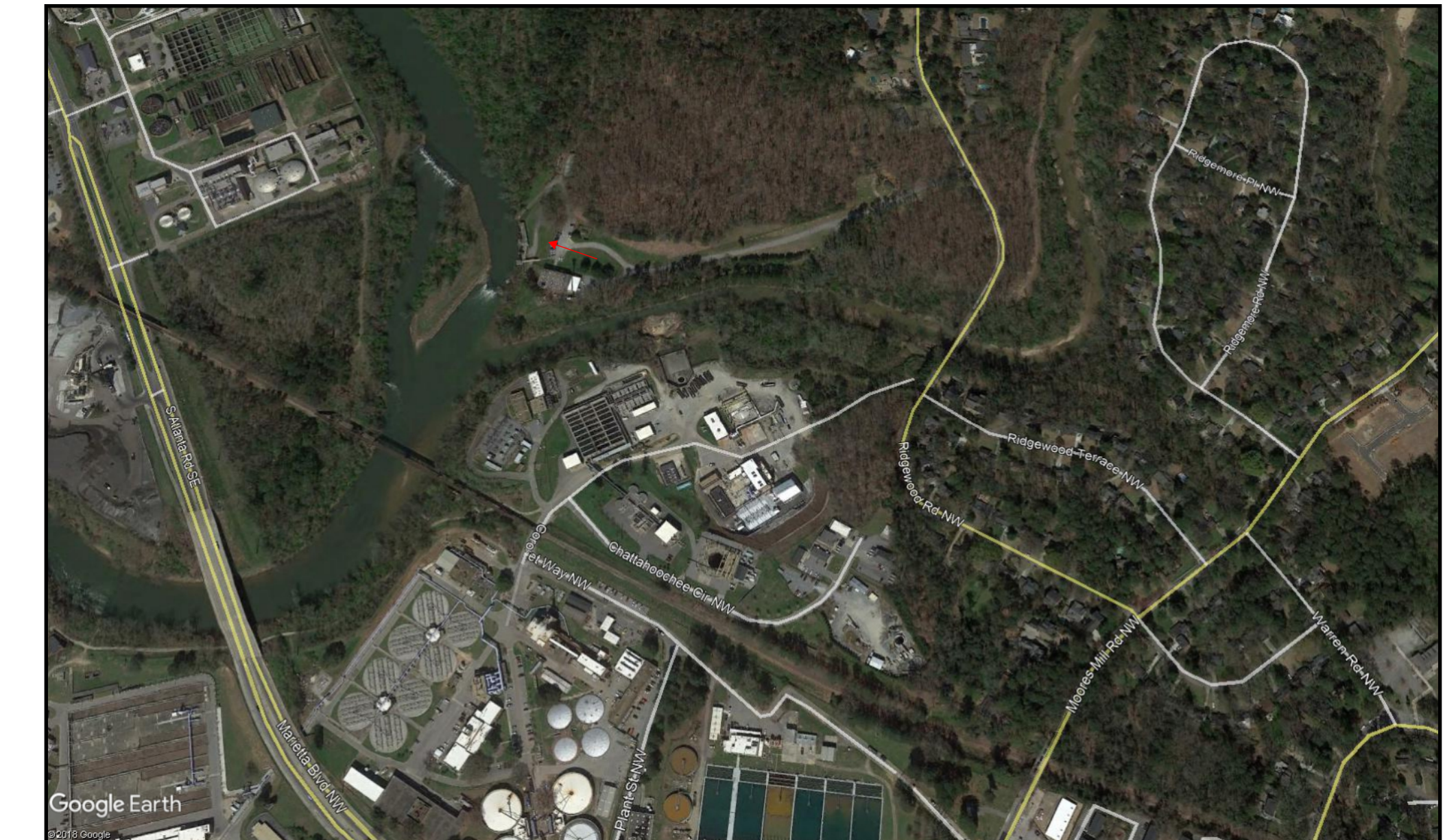
RIVER INTAKE PUMP STATION NTS 2566 RIDGEWOOD ROAD NW, ATLANTA, GA 30318 FULTON COUNTY
