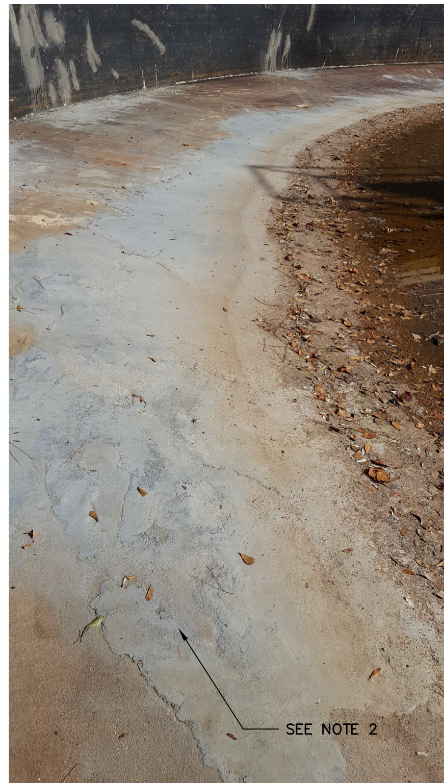
PHOTO 3: TYPICAL FLOOR SLAB
