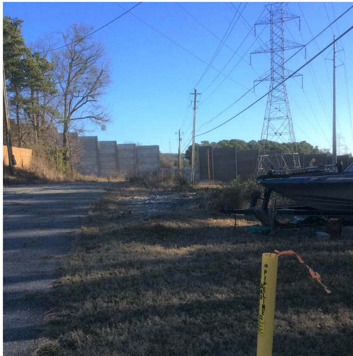
Photo 01: ROW – Barnsmill Road @ Beech Street AGL test station (galvanic system).
