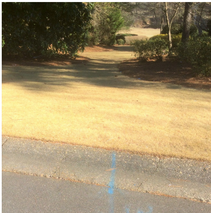
Photo 6: ROW – Creekwood Drive – Existing Water Pipeline
